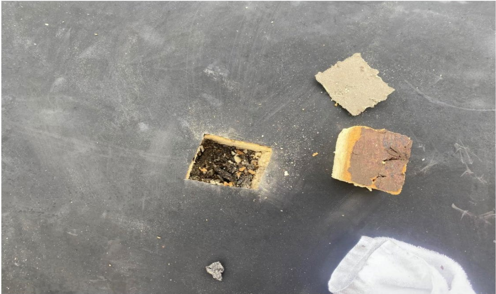
Roof Area A Test Cut
