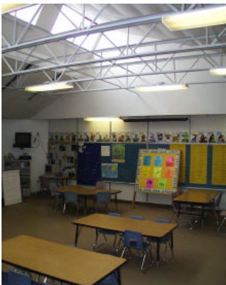
South Facing Monitor Skylights
