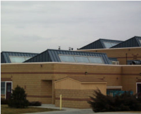
New School with Monitor Skylights
