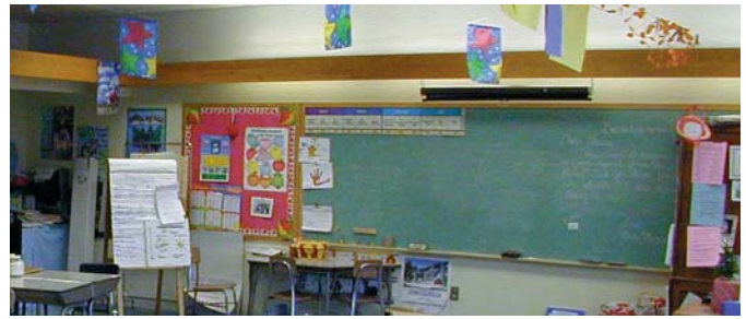
Valances (Type H) are an inexpensive way to light focal walls, but don't provide the best uniformity.
