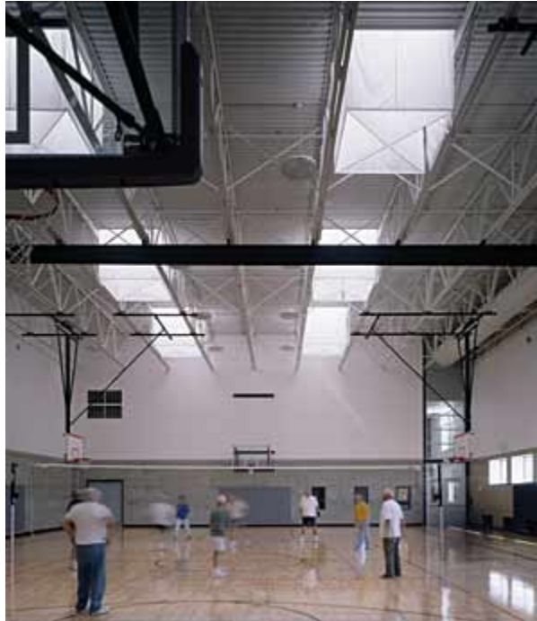
Southwest Community Center Gymnasium, Seattle, WA This gymnasium uses fabric skylight baffles to diffuse glare and make electric lighting unnecessary during daylight hours. Architect: Weinstein A|U . Photographer: Jamie Myers Forsythe
