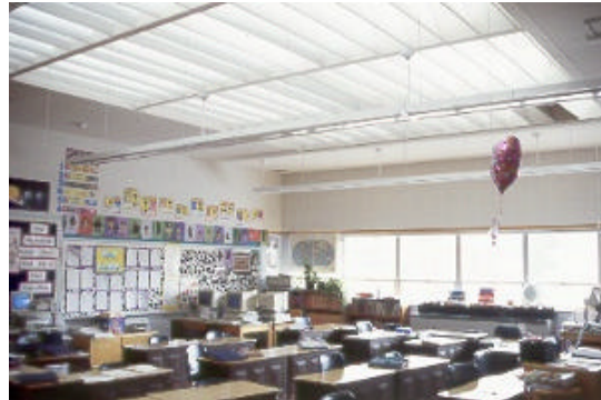
Central Skylight and Diffusing Louvers
