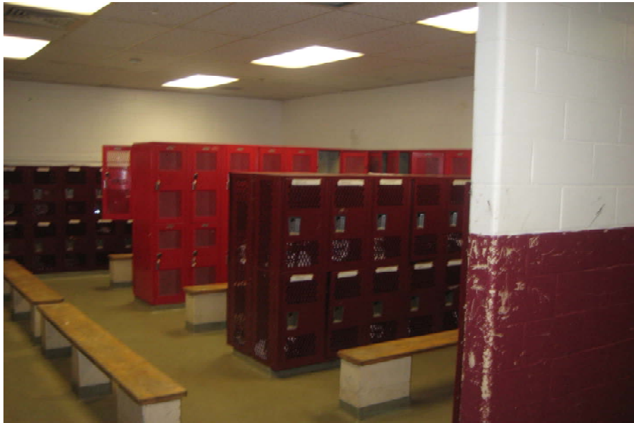
Inadequate Locker Rooms
