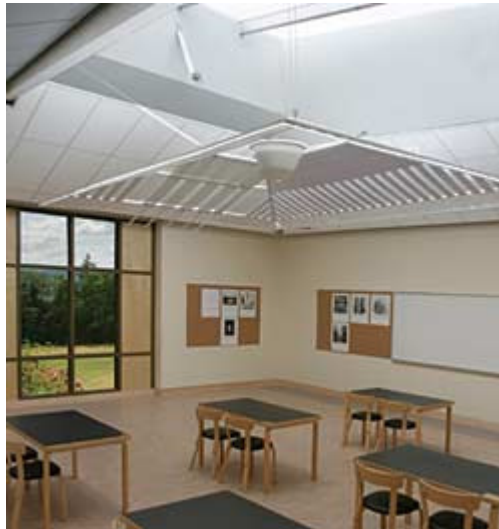
Mt. Angel high performance prototype classroom, Mt. Angel, OR: A rectangular suspended device dubbed “the halo” is made of translucent material that reflects part of the light onto the ceiling and walls, while letting part of the light into the room. Design team: BOORA, SOLARC, Prof. Charlie Brown of the Seattle Daylighting Lab, and SRG Partnership
